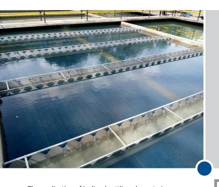
The application of inclined settling planes to increase the sedimentation performance is an unchallenged technology; it's applied in numerous plants worldwide covering hundreds of applications.
